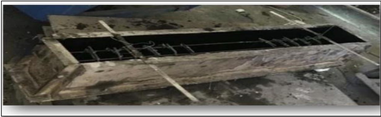
Fig.5. beam specimen mold during casting.
