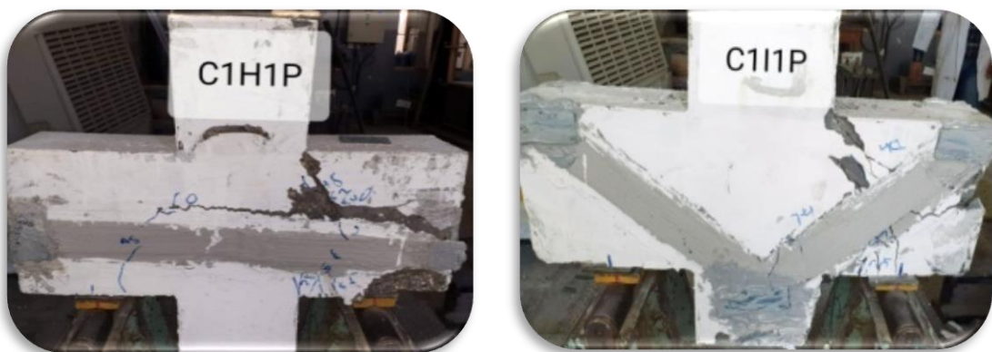
Plate(4) Crack pattern of strengthened corbels (C1H1P, C1I1P)
