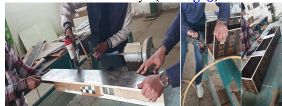
Fig. 3 Preparing the Beam Molds.
