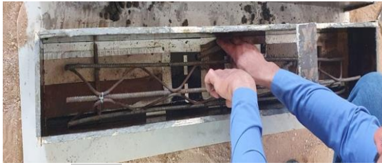
Fig. 5 Reinforcement of Steel.
