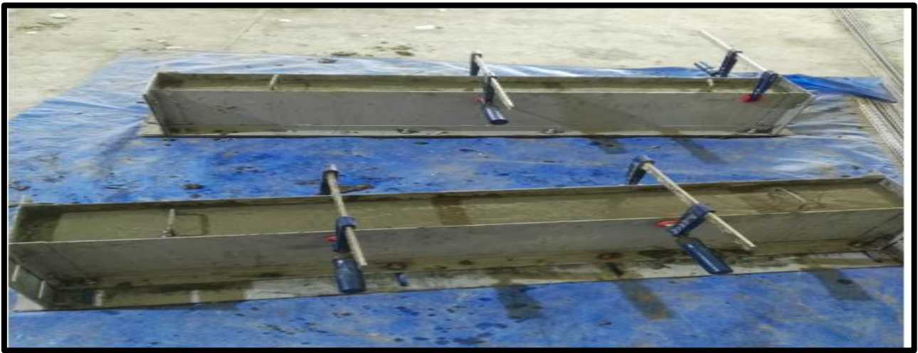
Fig.2: Casting of RC Beams
